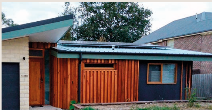
Reclaimed timber from the original house, finished with Organoil, is used as a feature on the home. On the right, is the blue-painted Shadowclad—the decorative timber features look good, but make repainting more difficult.
