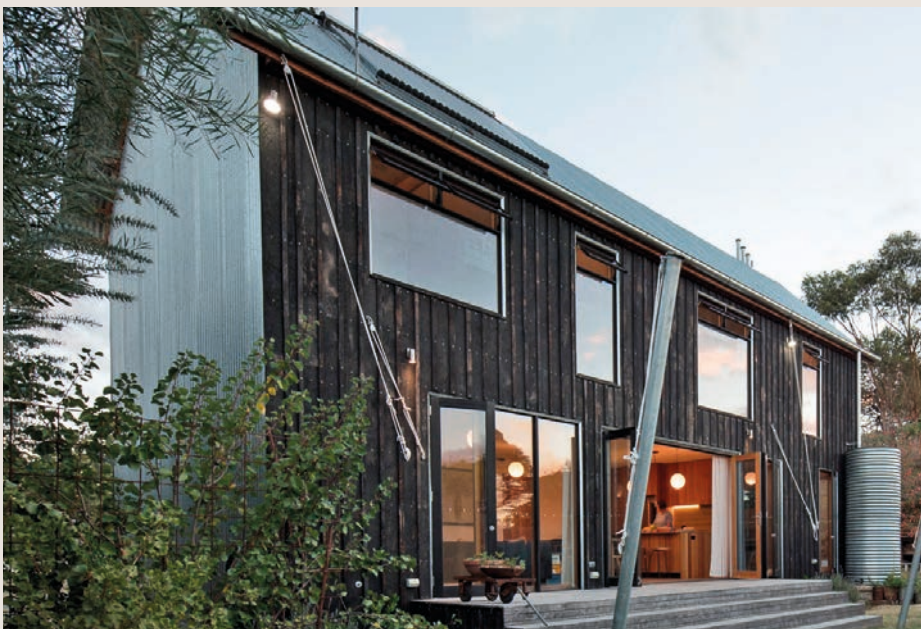
Quentin used charred timber cladding on his own house in Victoria, along with Z600 galvanised steel for long life.
