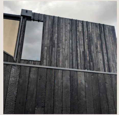
Charred and oiled timber on another of Quentin's projects (designed by Chiverton Architects), about 18 months after install.
